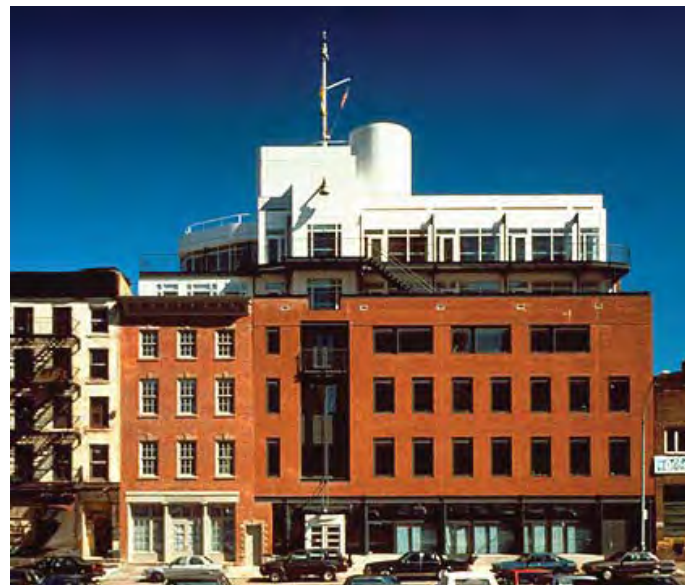
Setbacks above the street wall can provide space for rooftop terraces that take advantage of views to the waterfront
