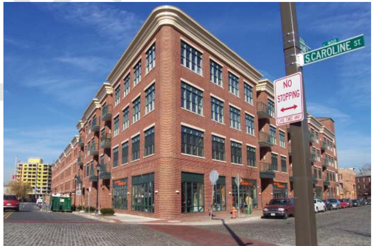
Parking at key locations should be screened or wrapped by other uses.
