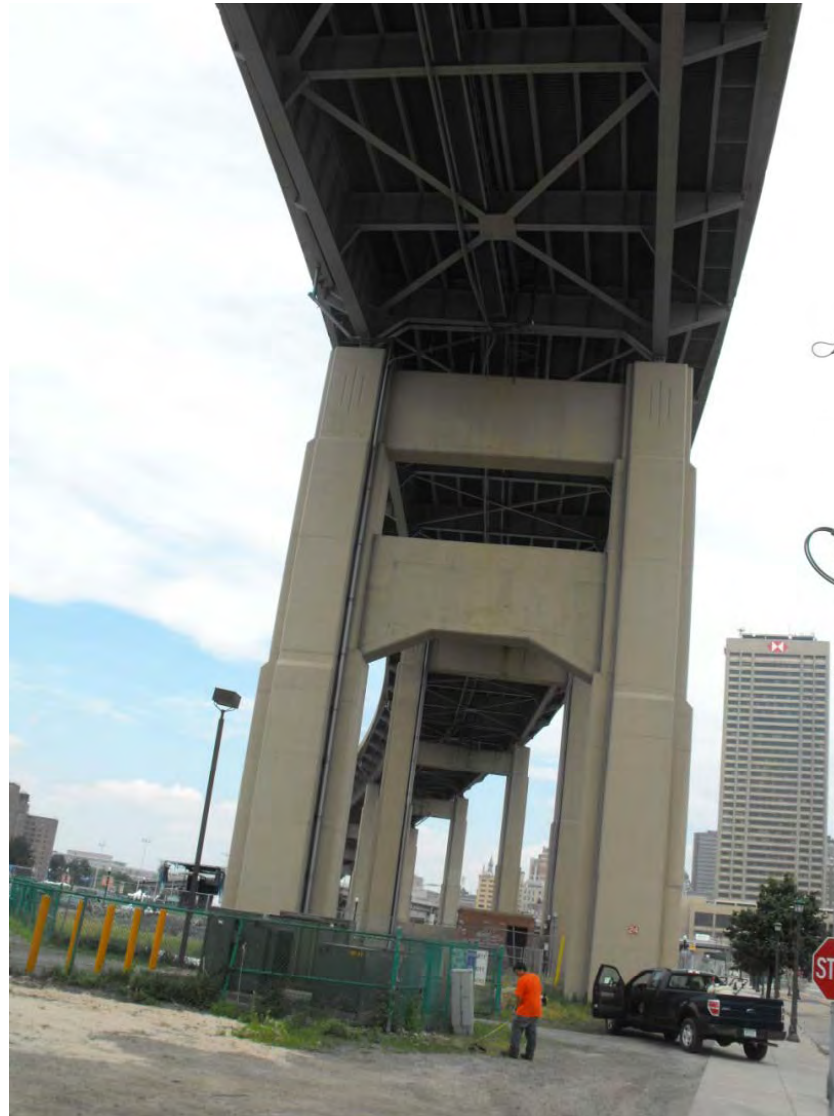
Under Skyway, facing north
