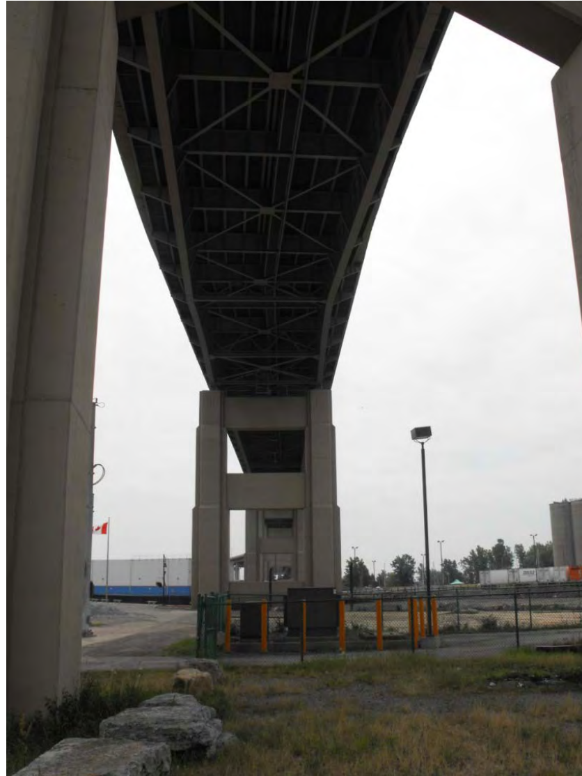
Under Skyway, facing south
